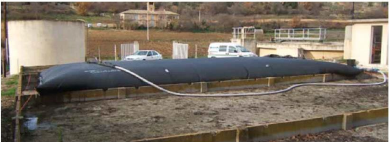
Plate 4.1 Example illustration of geotube being filled
