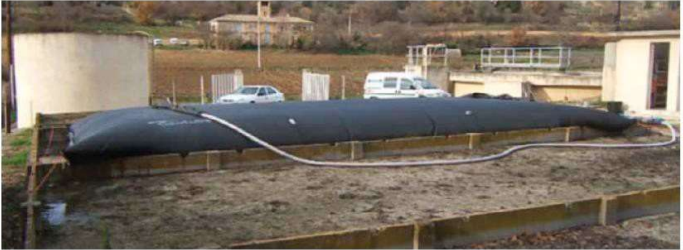
Plate 4.1 Example illustration of geotube being filled
