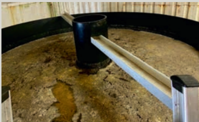
Figure 2. In this image the sludge in tank 4 can be seen. Because the active sludge was used with salt water from the RAS, the sludge is floating. Other methods to take out the sludge are needed compared to treatments for fresh water where the sludge settles at the bottom.
