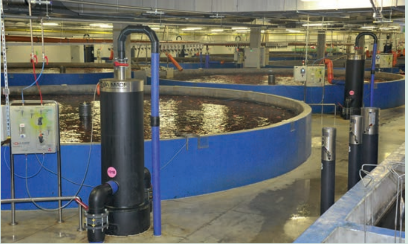
Recirculation aquaculture systems are complex and require trained personnel to manage them, but they allow adjustments to be made to all the parameters within the system.
